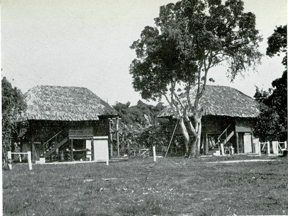
Experimental staff housing at Carimagua built largely from native materials.
