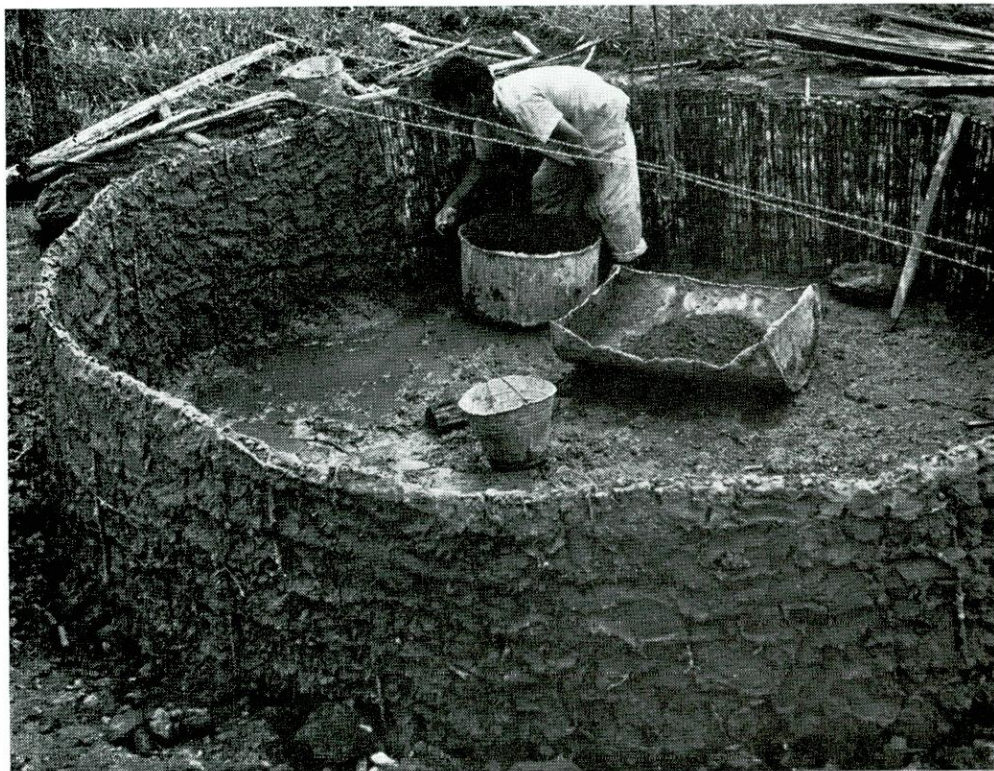
A water tank takes form over base of palm sticks wired together with used barbed wire. No forming lumber is required.
